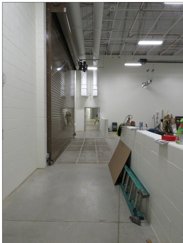
Pictured far left is a cell in the general population area. The photo at left shows the new Sally port which connects the new jail to the Judicial Center for secure inmate movement. Below left is the new intake area. Below are new cells. (Brad Jennings photos)
