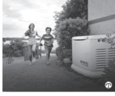
**A permanently installed home standby generator can power the home for extended outages, running on natural gas or propane.**
