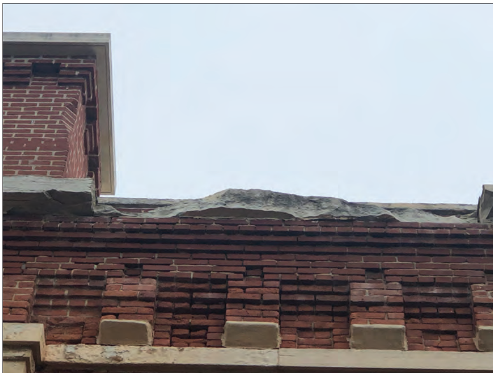
The Amboy Depot Museum Committee is moving forward with a rehabilitation and restoration project on the depot. Above, is a picture of some of the concrete cornice that is crumbling.
