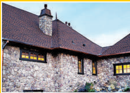
STONE, SIDING & ROOFING
