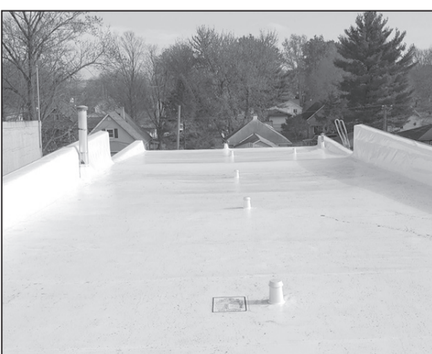
Northern Illinois Seamless Roofing, Inc. specializes in flat and low slope commercial roofing by installing the Duro-Last family of roofing systems. Duro-Last is the world's largest manufacturer of pre-fabricated single-ply roof systems. This system is ideal for any flat or low-slope roof.
