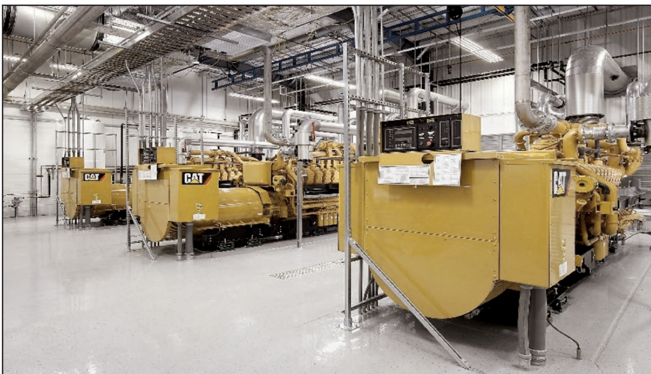
The power plant collects greenhouse gas from the landfill and cleans it before sending it to three large Caterpillar engines that run off methane gas and produce energy.
