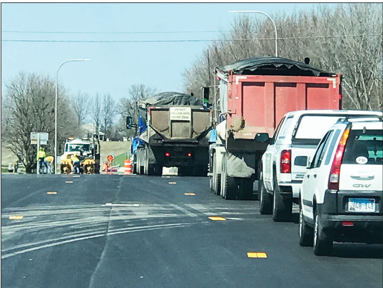
Road work ahead Traffic is backed up on Route 251 in Mendota as a road construction crew works on refinishing the roadway. Work includes road milling and resurfacing, and reconstruction of ADA sidewalk ramps. Traffic will be controlled by flaggers when workers are present and side streets may occasionally be closed for short periods of time. Motorists can expect delays and should allow extra time for trips through this area, and be prepared for slow and stopped traffic. This $1.9 million project is anticipated to be completed by the end of summer. (Reporter photo)
