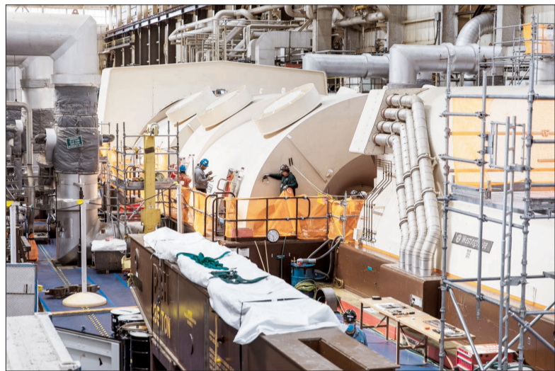
Workers inspect the Unit 2 generator at the Byron Station.
