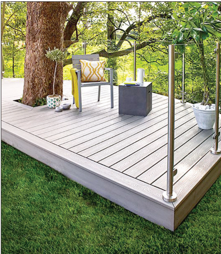
Due to its low profile, a ground-level deck doesn’t typically require safety railings or stairs, so the costs are comparatively lower than building an elevated deck in terms of both materials and labor.
