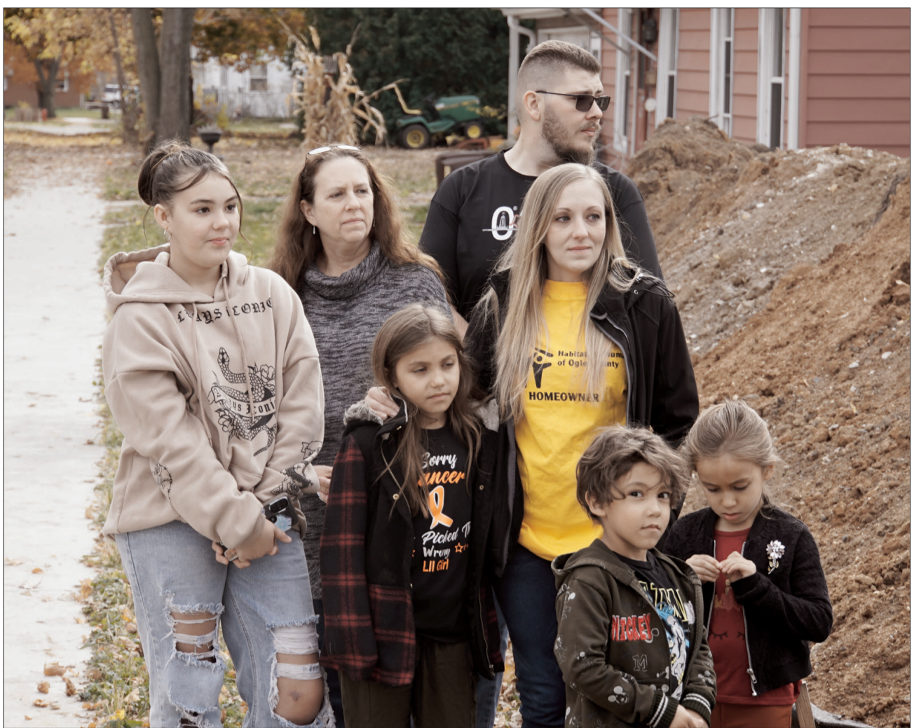
On Sunday, Oct. 30, a groundbreaking event was held by Habitat for Humanity of Ogle County for its latest home in Rochelle.
