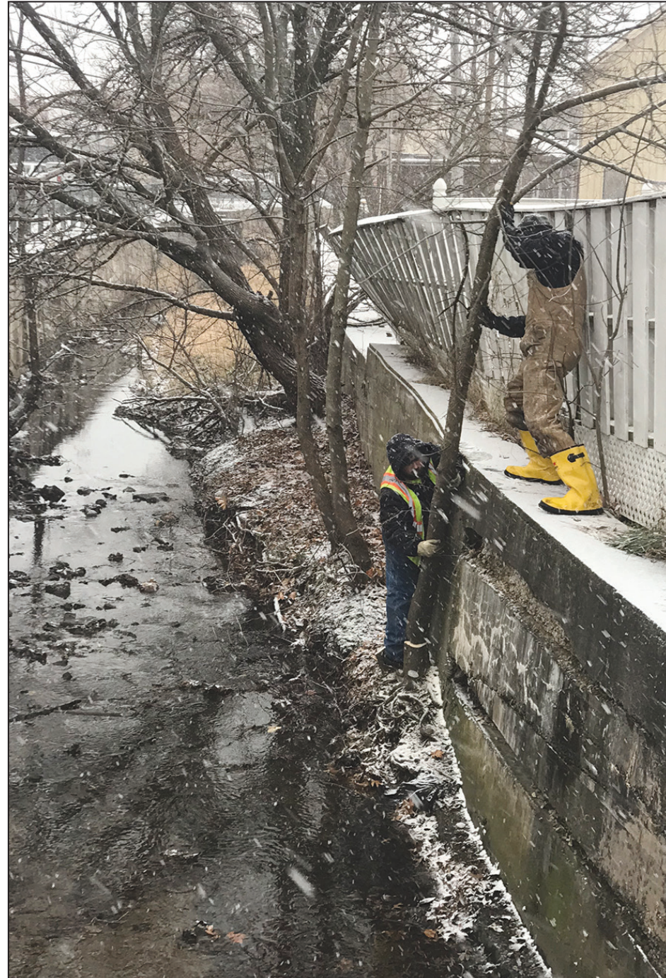
The Mendota Garden Club and the city of Mendota recently teamed up to clear small trees and brush from Mendota Creek to preserve the integrity of retaining walls and also to enhance the flow of water in the creek. Working in a section of creek between Jefferson and Monroe streets are Steve Lauer of the Mendota Garden Club, right, and Ethan Guelde of the city.
