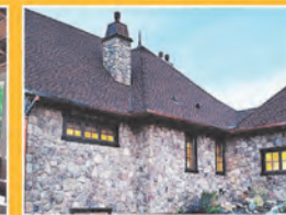
STONE, SIDING & ROOFING
