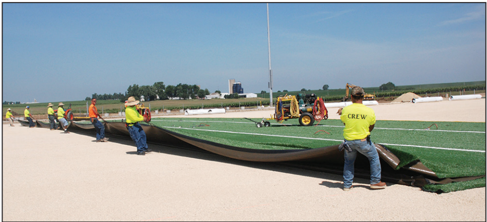
Workers stretch the field turf into place at the MHS athletic stadium in July 2011. The original turf will likely be replaced within the next three years.
