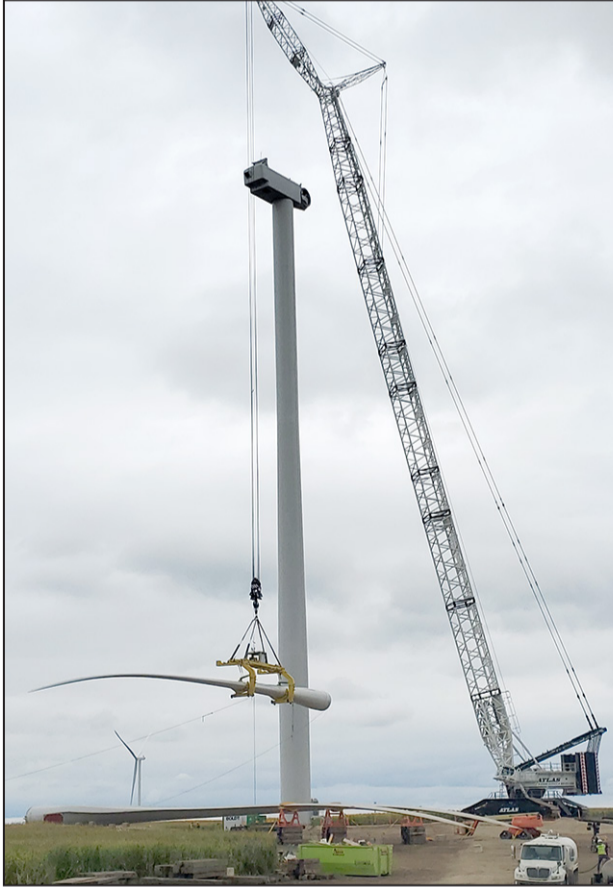
A blade is taken off of a wind turbine during the repowering process at the GSG wind farm north of Mendota. (Reporter photo by Brandon LaChance)
