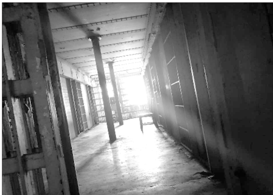
Inside the hallway at Historic Gila County Jail.
