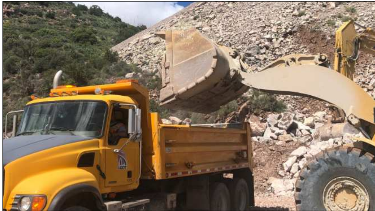
ADOT trucks work to repair US 60.
