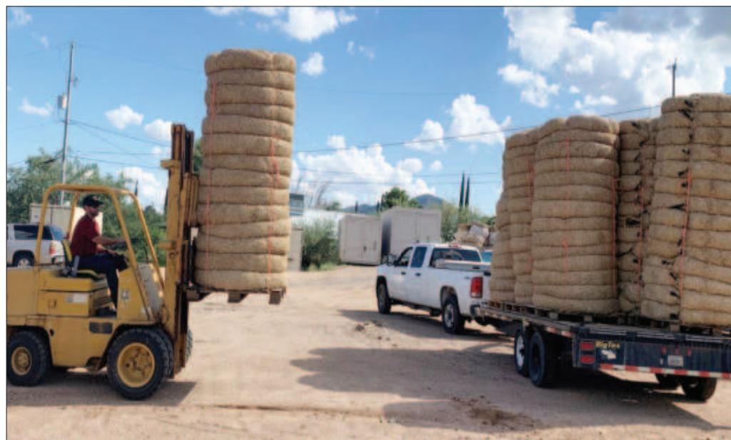
A Globe Ranger District employee uses a forklift to unload straw wattle. Pinto Valley Mining Corporation delivered 7,000 linear feet of straw wattle to the district for future installation at the Ellis Vein Mine site.
