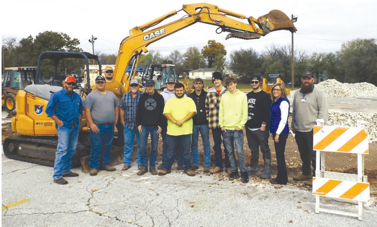
Members of North Arkansas College's Heavy Equipment Program will be contributing to repairs at the North Arkansas Regional Medical Center's employee parking lot. CONTRIBUTED PHOTO
