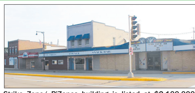
Strike Zone/ P'Zones building is listed at $2,100,000. Contributed photo.
