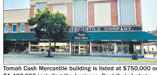
Tomah Cash Mercantile building is listed at $750,000 or $1,400,000 including the business. Contributed photo.
