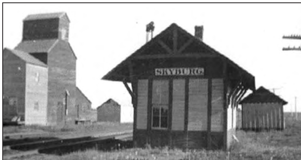
Skyberg train depot and grain elevator
