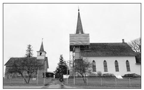
Valley Grove church steeple is enclosed by scaffolding and heavy plastic wrap so River City Builders & Millwork can repair water damage. Taking advantage of the mild winter, RCBMI's Jarrod Wood expects to finish the. \$200,000 repair by April.
