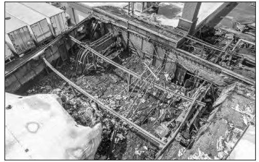
An overhead shot of the most severely damaged portion of the Hastings Creamery. The roof collapsed in this area as it was one of the hottest spots in the fire. This is where a good portion of the production was done at the plant. For reference, the photo through the side door is through the closed door on the upper portion of this image.
