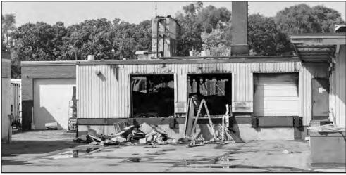
This loading dock was primarily used by trucks returning to the creamery with empty crates when the creamery was in operation. As you can see from the image, there are piles and piles of cardboard boxes on the docks that added to the fuel for the fire.
