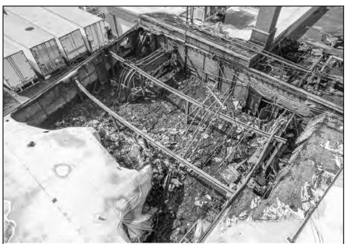
An overhead shot of the most severely damaged portion of the Hastings Creamery. The roof collapsed in this area as it was one of the hottest spots in the fire. This is where a good portion of the production was done at the plant. For reference, the photo through the side door is through the closed door on the upper portion of this image.
