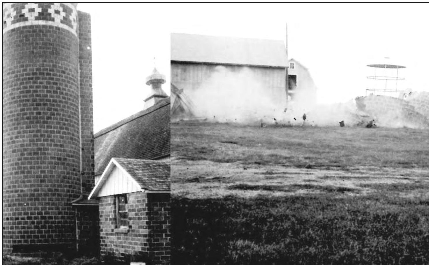
The 60-foot-high silo on the Kleven farm north of West Concord had aged out and was knocked down in the summer of 1966. Emery had then lost his target for hitting towering home runs.
