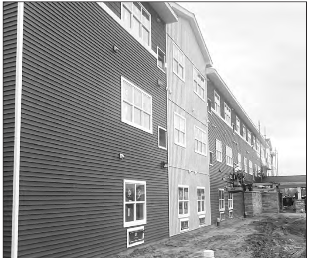
Exterior of building nearly complete
