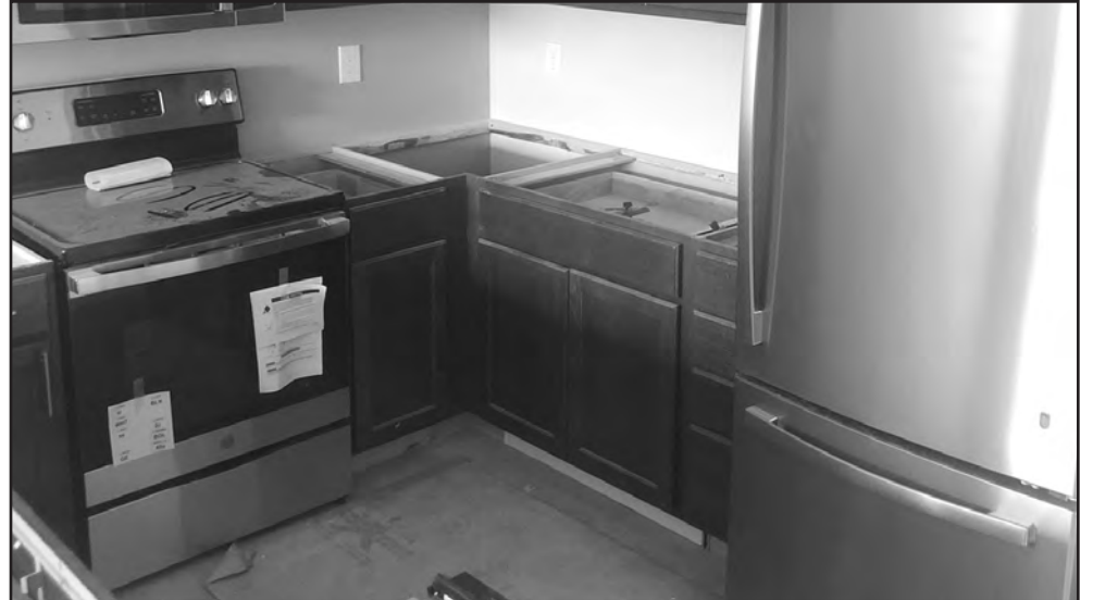
Beautiful woodwork in kitchens and appliances are being installed!
