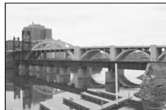
The Robert Street Bridge, St. Paul, designed by Toltz, King, and Day and also on the National Register.
