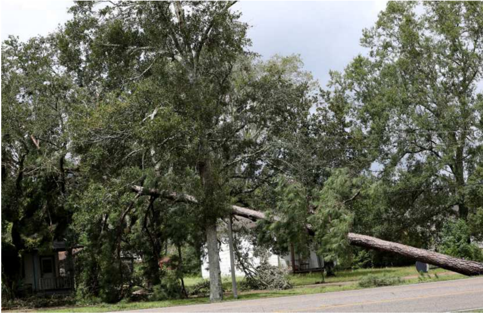
A tree is atop a house in the Town of Livingston following Hurricane Ida , which struck the state on Aug. 29, 2021.
