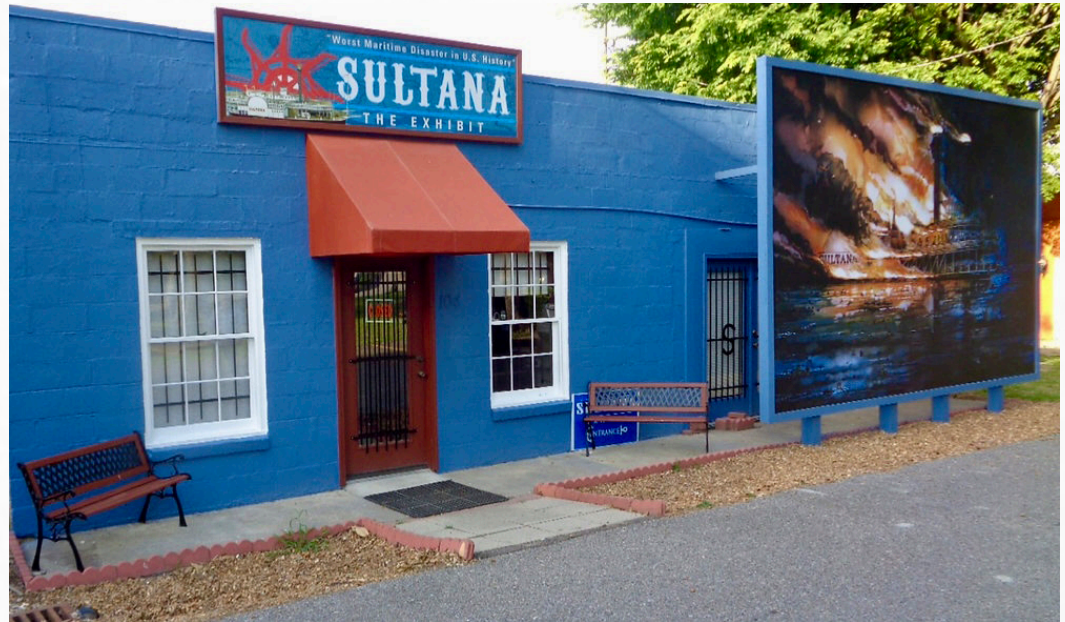
The Sultana Disaster Museum located in Marion, Arkansas.
