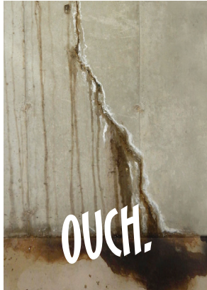
Wall Cracks
