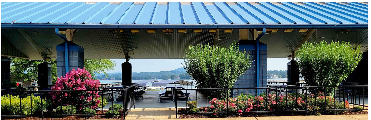
Balboa Pavilion Project.
