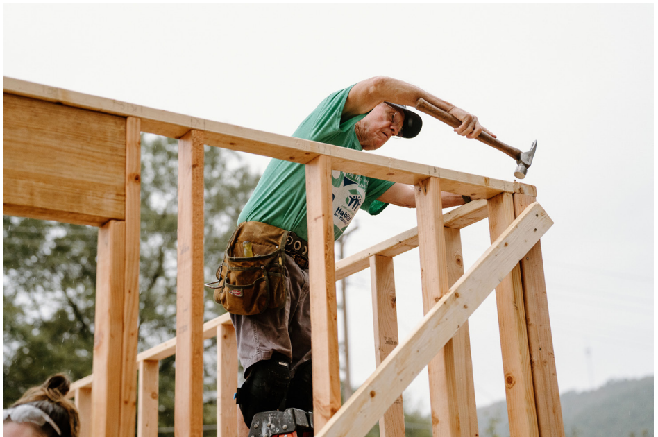
Framing a wall in a recent build.
