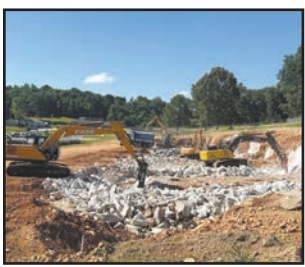
Robotics Center construction Page A3
