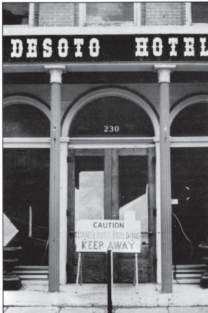
The front of the DeSoto House Hotel during the renovation 40 years ago.
