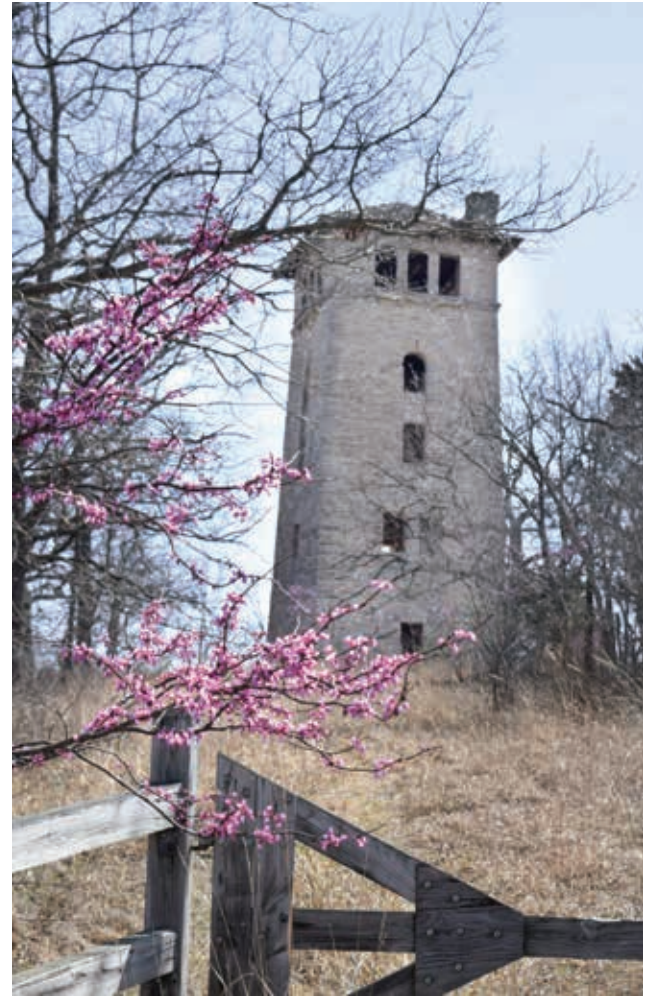
The five-story-tall water tower was built with sandstone brought to the construction sight by mule-pulled iron carts on tracks from the property's quarry.
