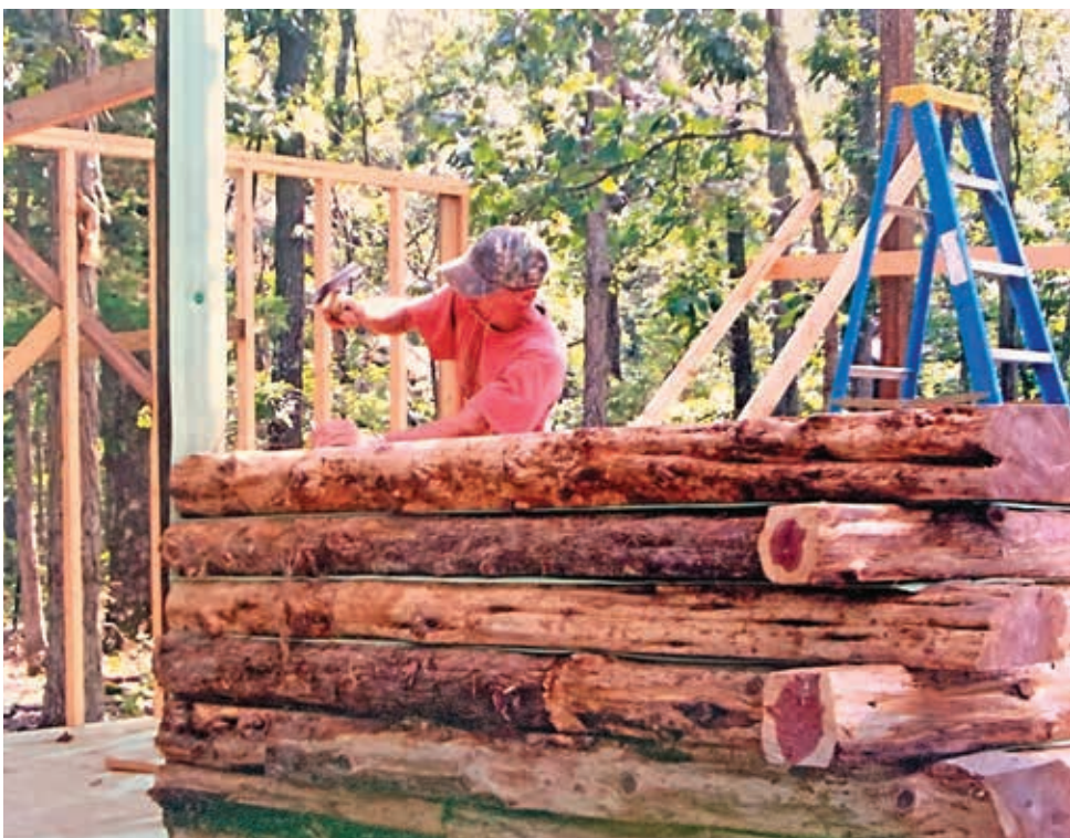
Ronnie Wilson working on nailing the logs in place. CONTRIBUTED PHOTO
