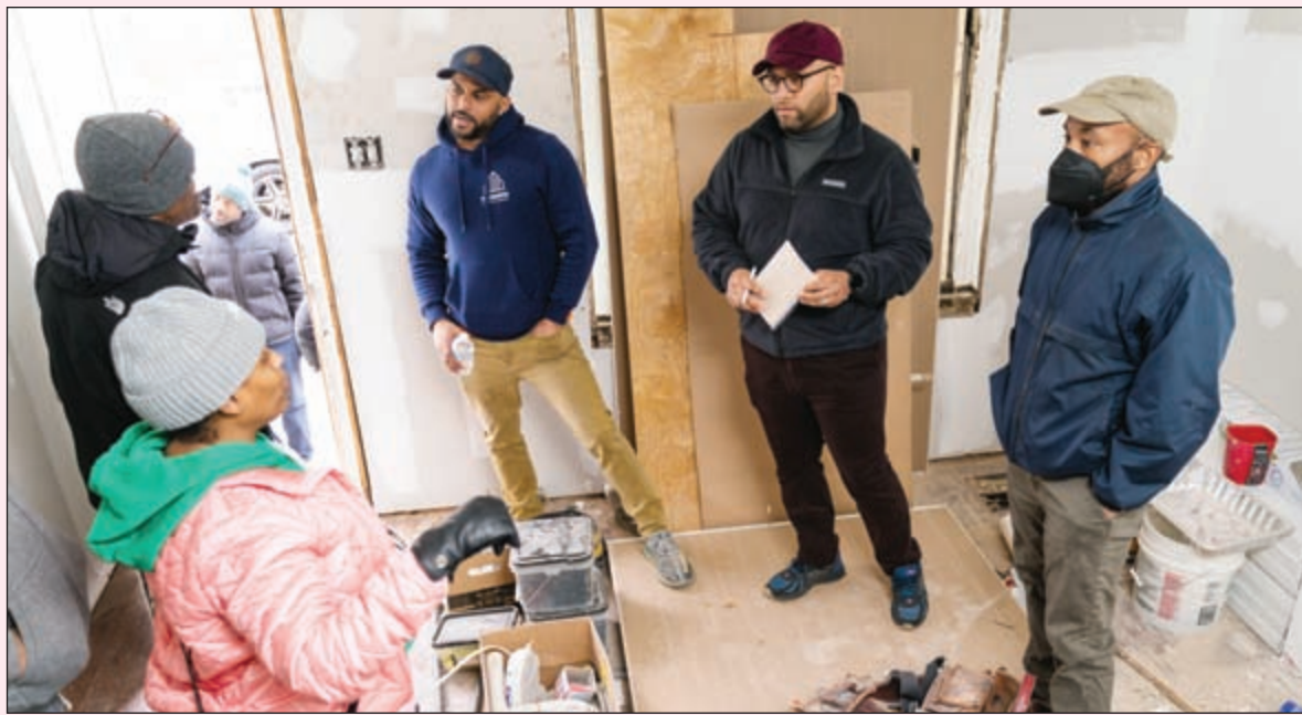
Jumpstart graduate Rhakeim Miller (picture in the center with a red cap and glasses) walks through a construction project as part of the coaching program. Photo by Chris Baker Evens.
