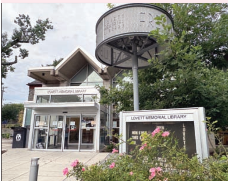
Lovett Library's six-year-old HVAC system was causing humidity issues that forced the building to close periodically this summer. It cost $21,000 to repair. Photo by Tom Beck
