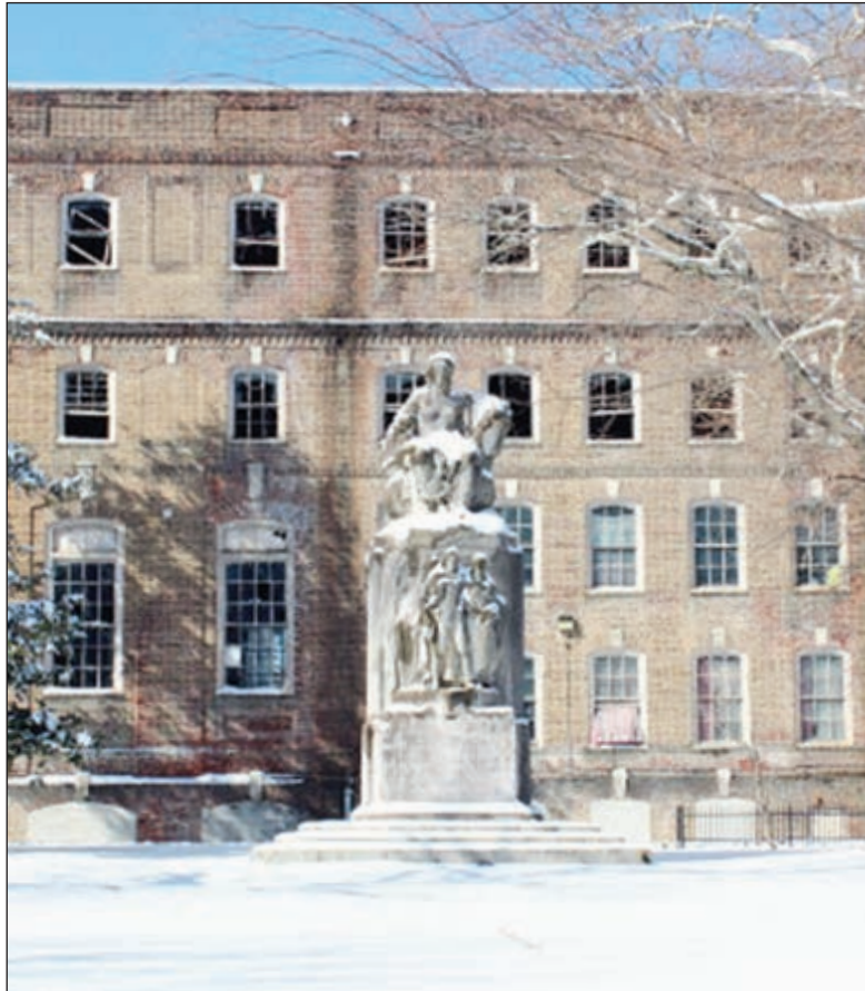
The Germantown YWCA, seen from Vernon Park.
