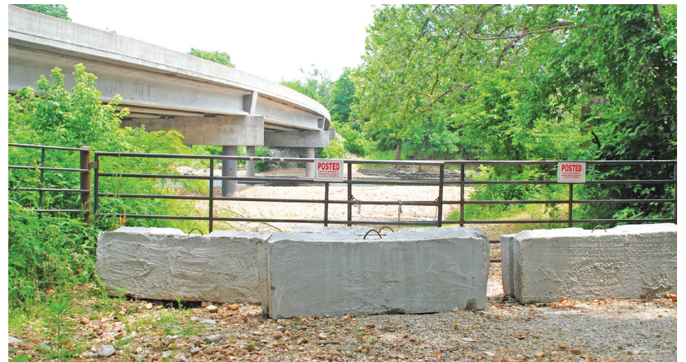
Gates and barriers stretch across a point on Canyon Road where river-goers once flocked to the Finley River at Lindenlure.
