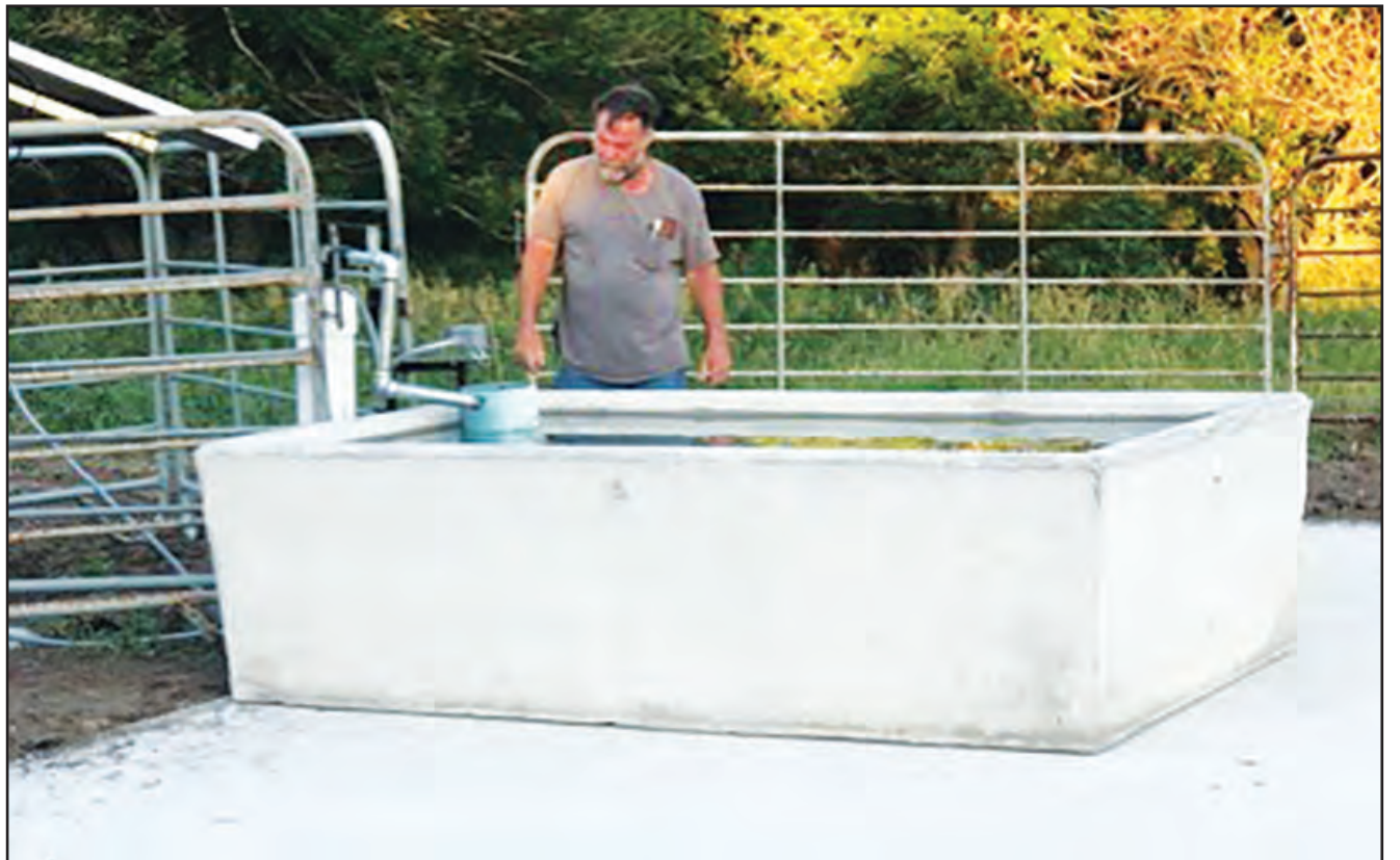
Erick Kadel stands by the solar well and pump, supplying a 600 gallon concrete stock tank. The pad of 18x22 feet, was poured before the tank was set on June 8, 2024. The solar panel is above on the fence to the left.
