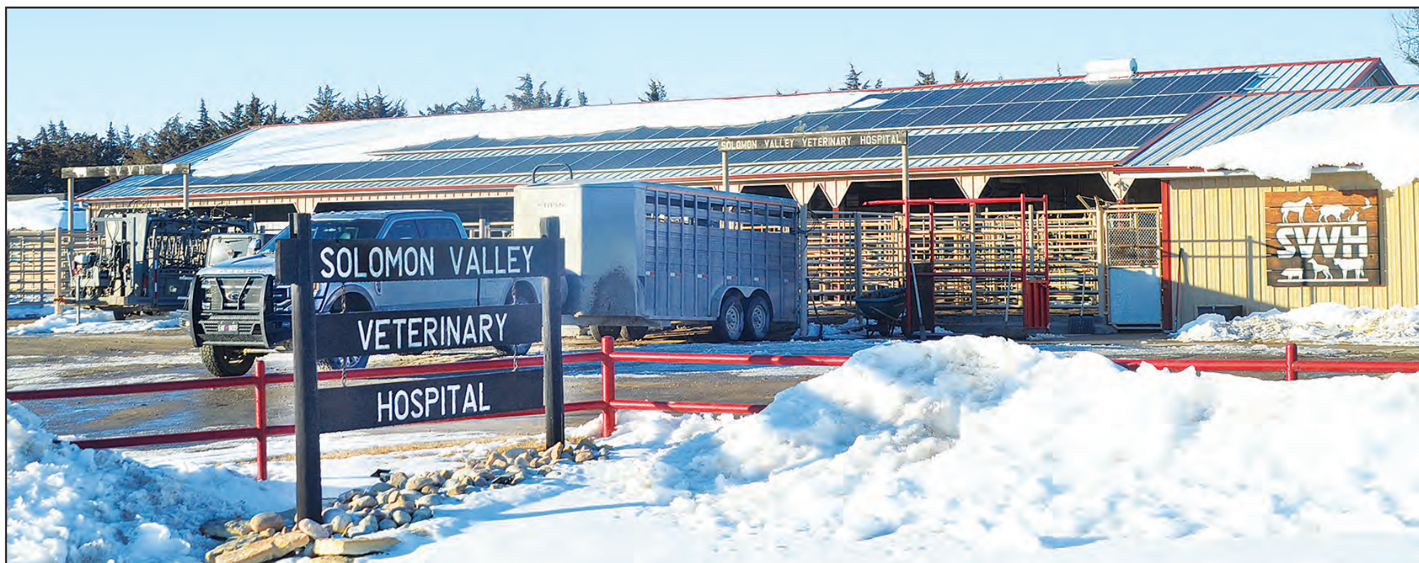
The Solomon Valley Veterinary Hospital have installed solar panels – as seen on the out building – to the entire clinic, and include the homes of Charles and Brady Luke as well.
