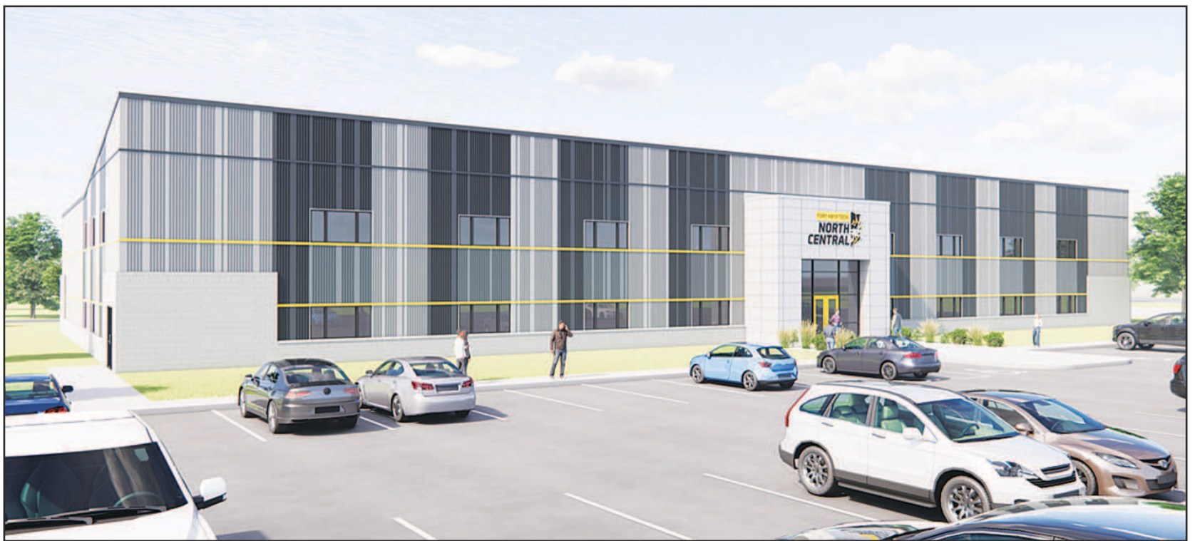
The new Construction Programs Building (under construction now) on the Hays campus.
