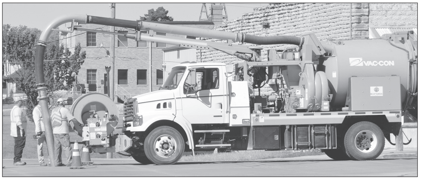
City of Beloit crews spent days working on cleaning the sewer systems.
