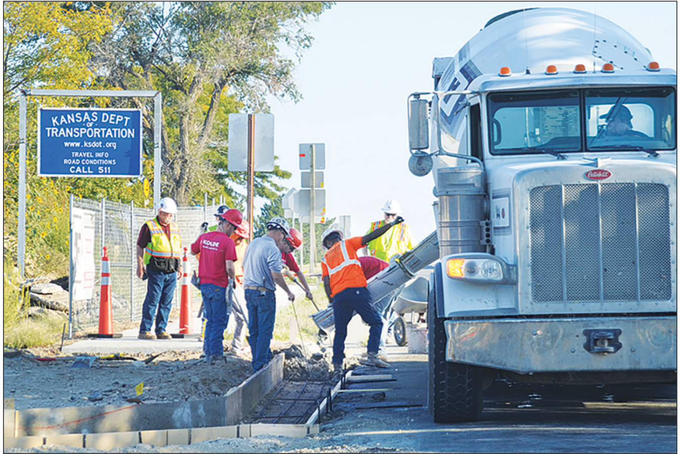
The KDOT building is put together, for the most part, and concrete is being poured by Abram's Ready Mix on Thursday for the curbside and sidewalk area along Independence and the 8th Street intersection in Beloit. SHARON SAHLFELD PHOTO
